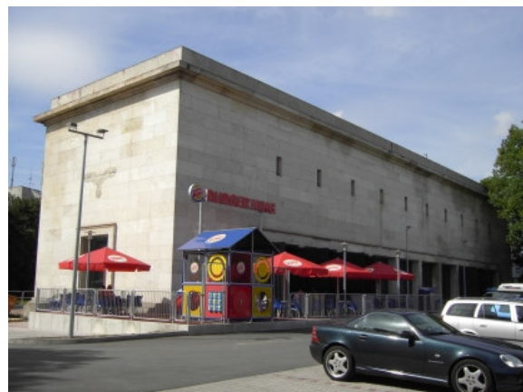
Power station for the Nazi party rallies at Regensburger Straße (see remnants of eagle to the left), now a “Burger King”
