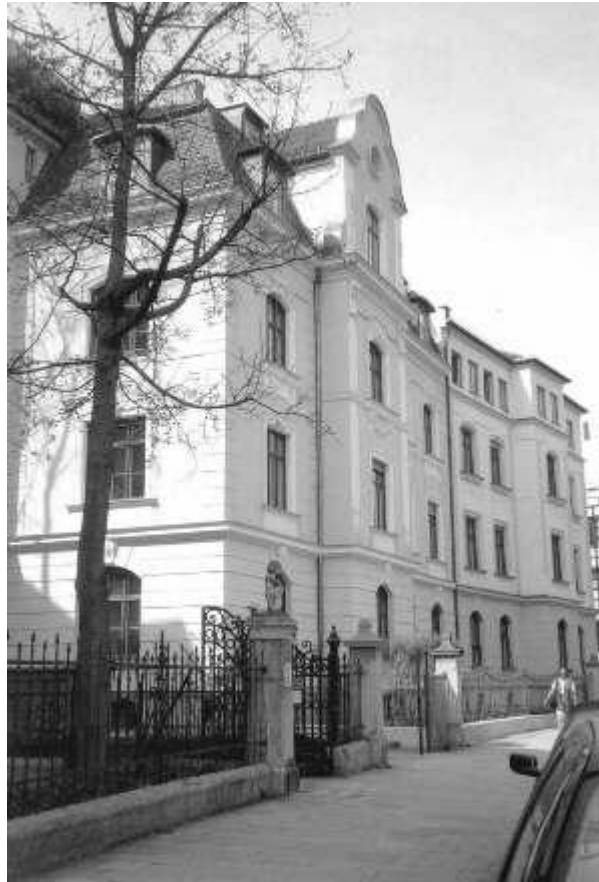
The residence of the Straus family: Kobellstrasse 13 (photo: Susanne Rieger)
